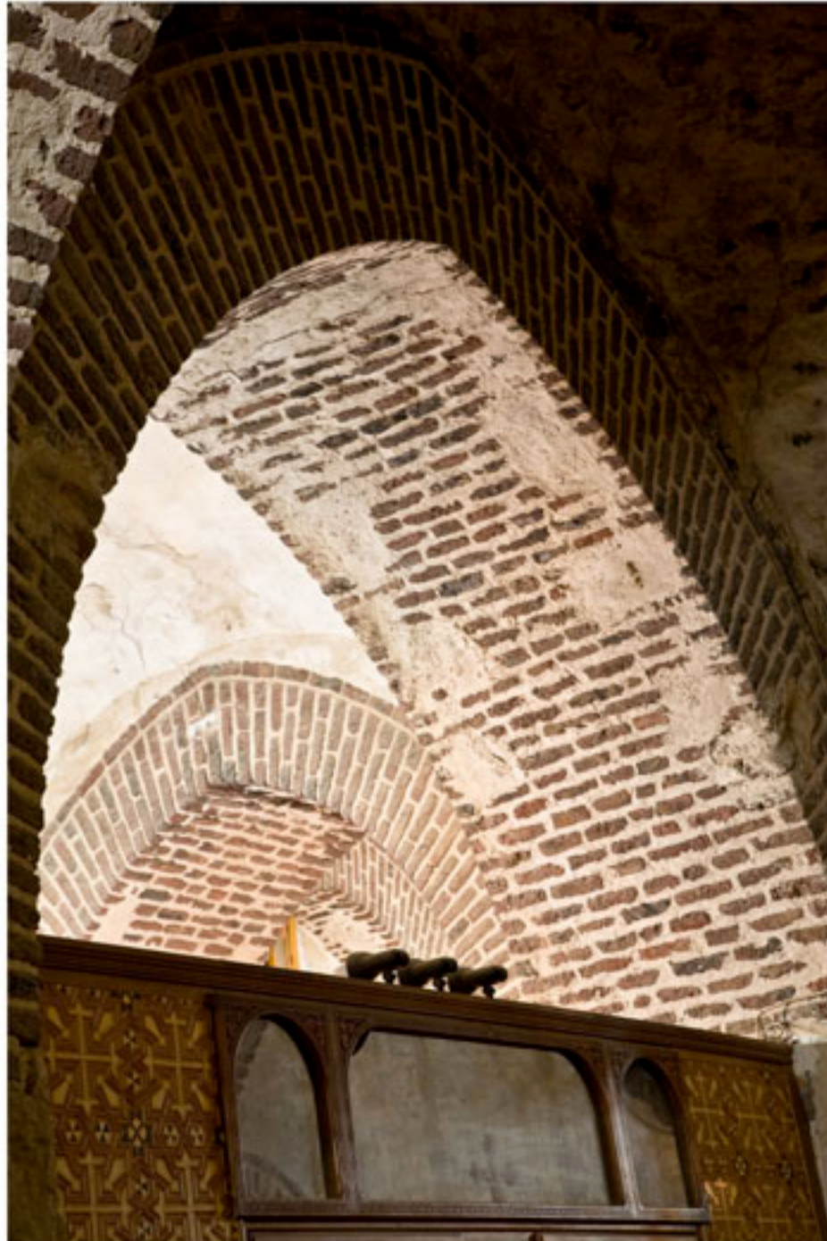
Arch detail in the Church of the Virgin Mary on the second floor of the keep (Area D).
