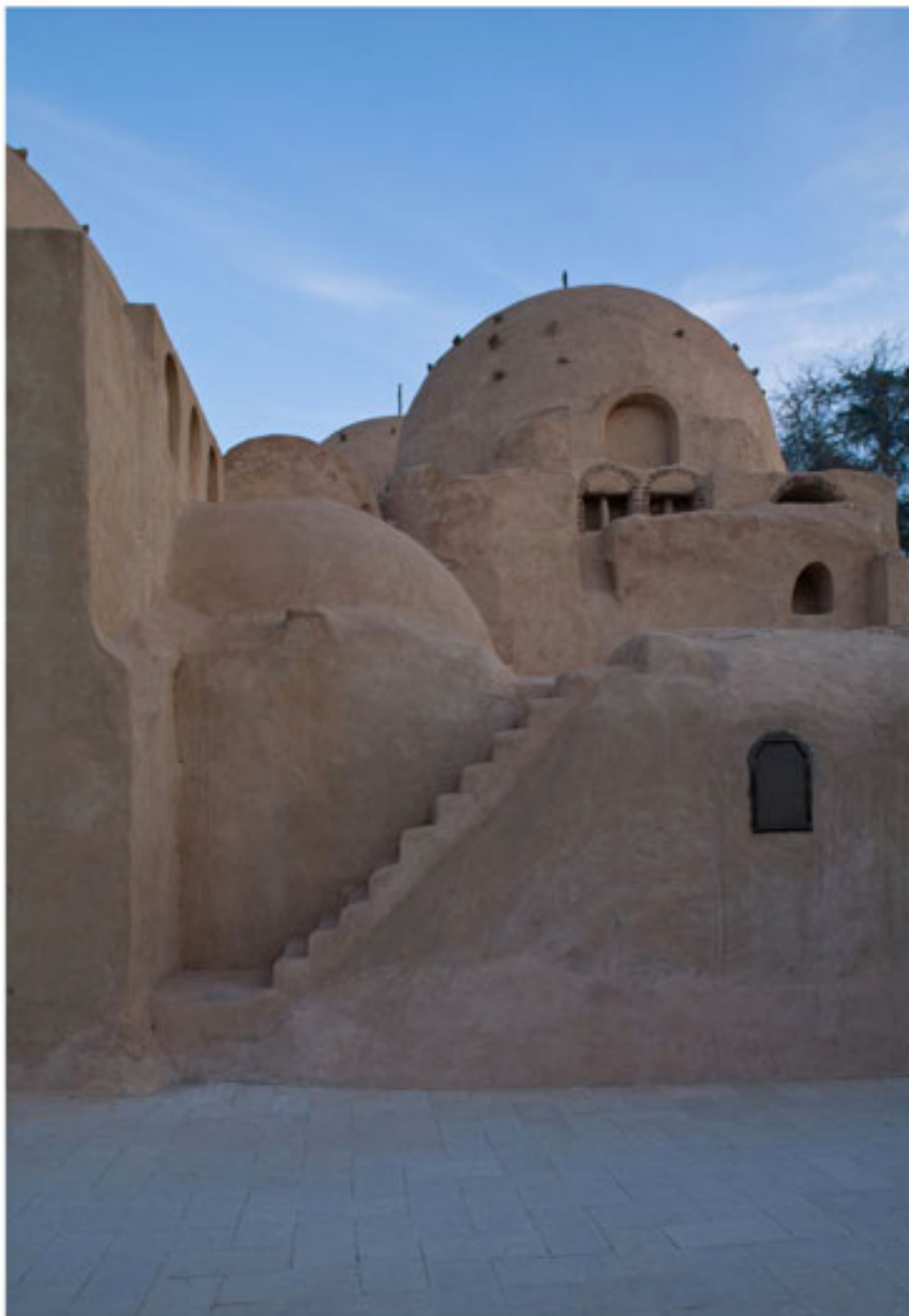
South wall of the Church of Saint Bishoy (Area H).
