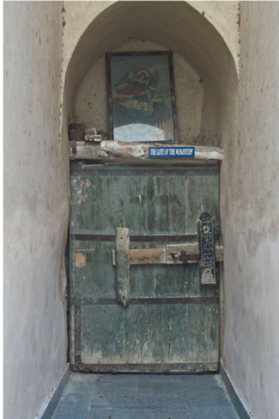
North door in north wall from the monastery interior (Area A).
